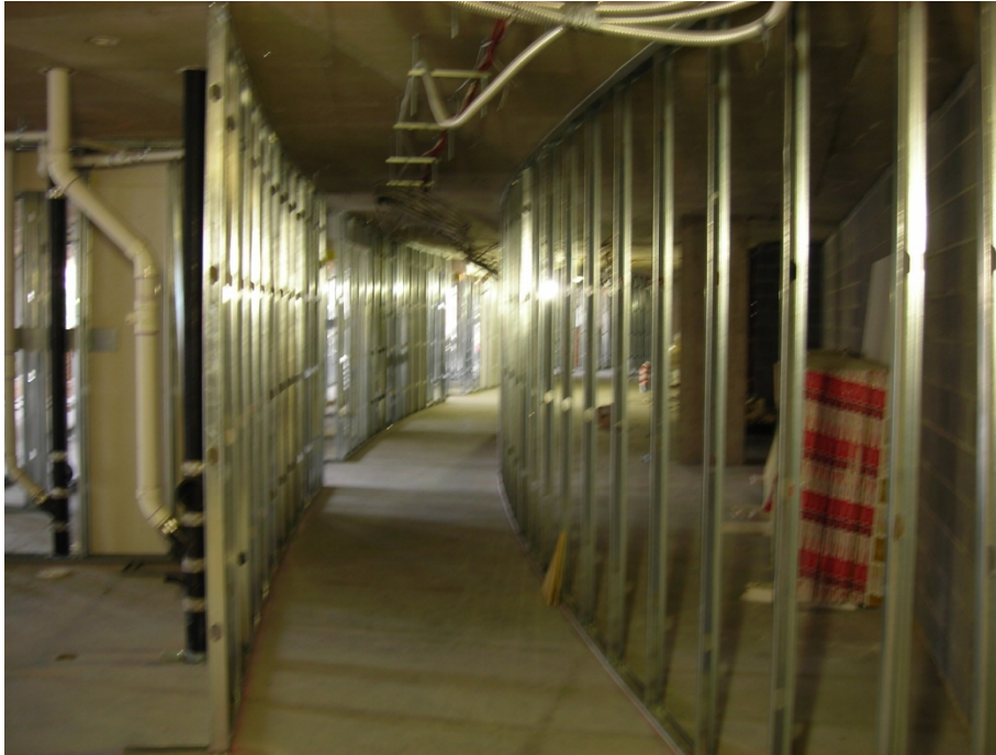
Photo 11: Interior view of a typical residential corridor.
