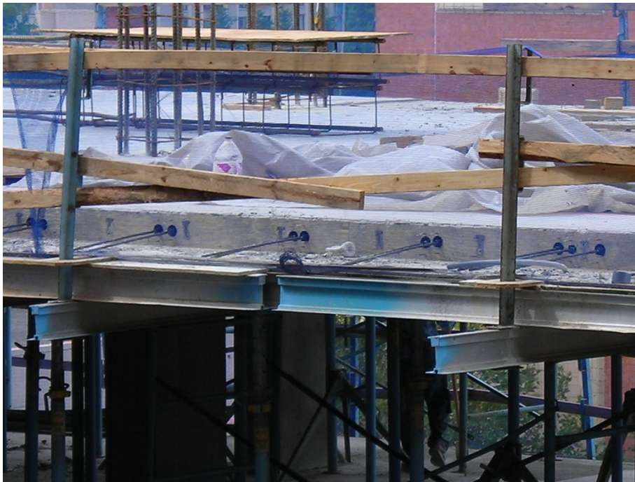
Photo 12: View of post-tensioning cables prior to jacking force application.
