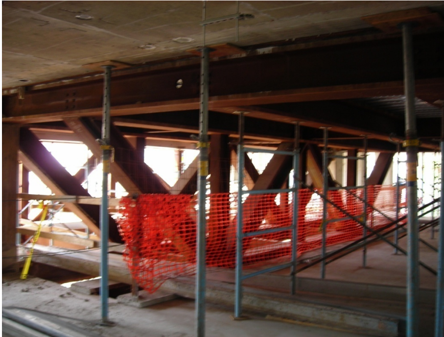
Photo 9: Interior view of pedestrian bridge steel structure.
