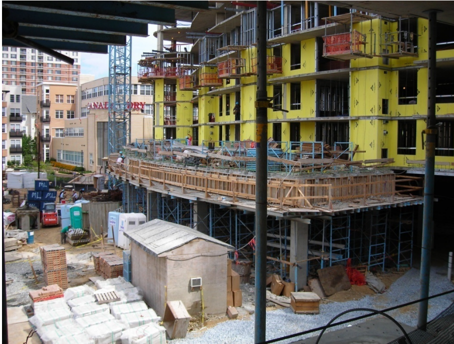
Photo 7: Partial view of lower floor construction on East-West Highway elevation (Southwest).
