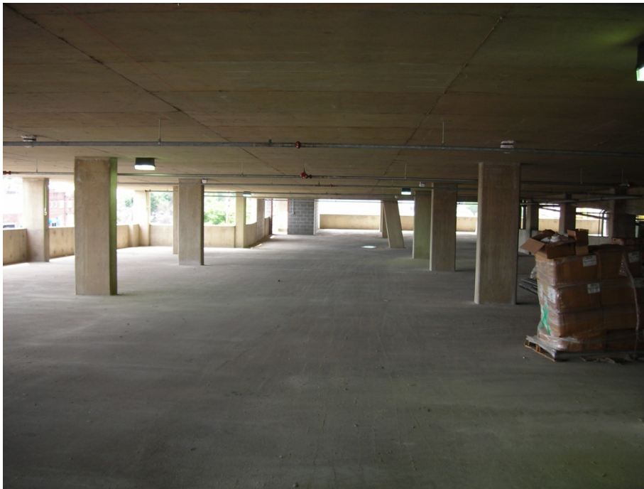
Photo 8: Interior View of the parking garage.
