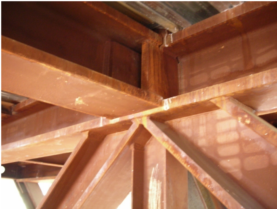
Photo 10: Typical full penetration welded connection of the bridge truss structure.
