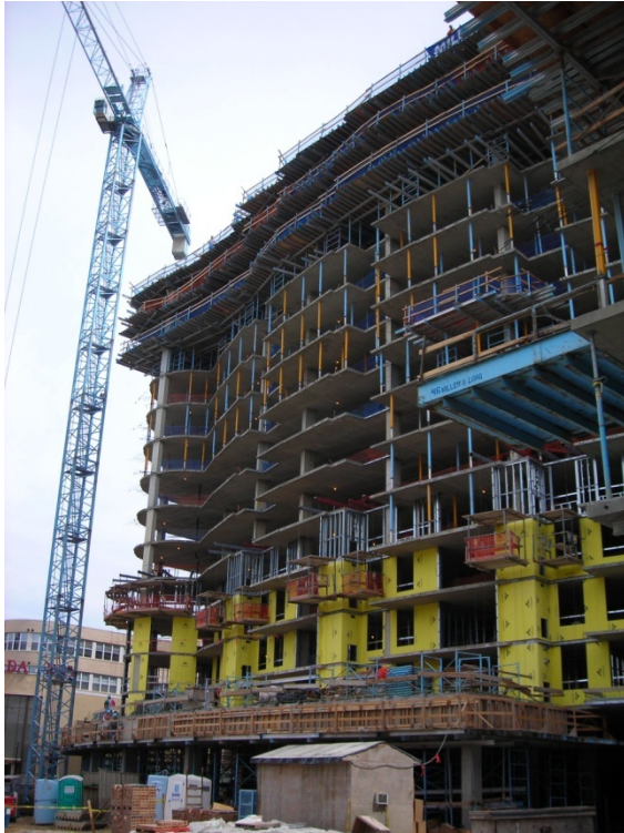
Photo 5: Partial view of the Southwest elevation.
