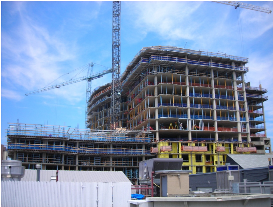
Photo 3: Overall view of Southeast elevation of Silver Spring Gateway.
