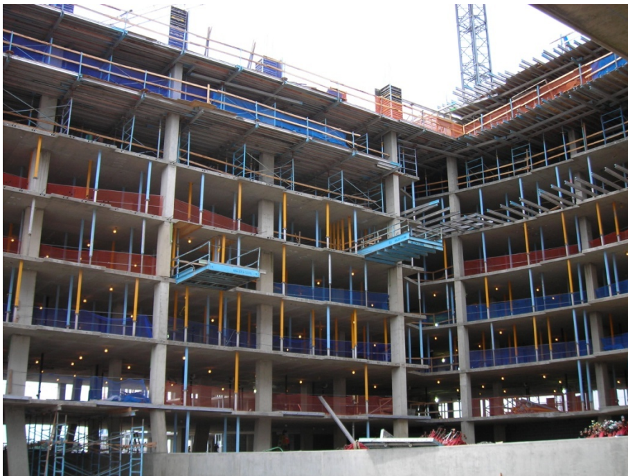
Photo 4: Partial view of courtyard from the top level of the parking garage.
